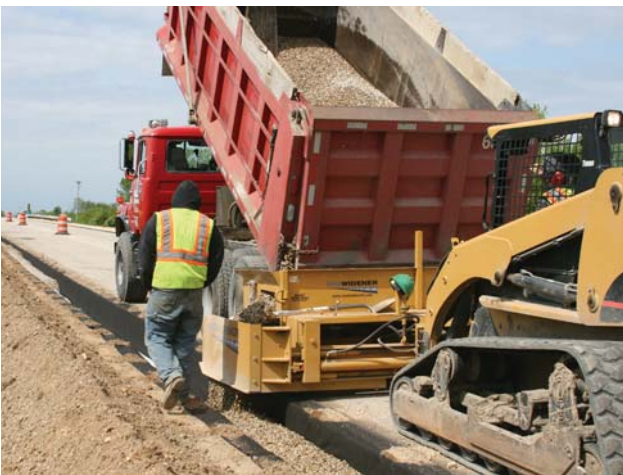
Trench backfilling with the FH Model.
